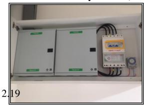
installed. Schneider brand is selected for main breaker box. A white cabinet is designed to cover the main breaker box for nice appearances.
