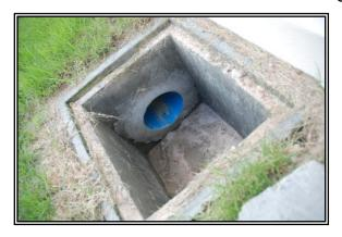
which is stronger and has longer service life than asbestos pipe even though the PVC is higher in cost.( <u>Remarks</u>: This is very important that the Project has to put forward since many
