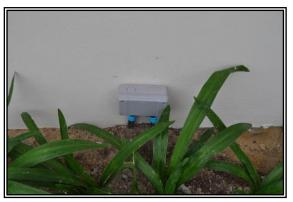
(Remarks: The Project decided to prevent termite problems in the long run by installing the termite extermination piping on the lower beams around the building of each house. This job will be done right after pouring concrete for lower beams. House will have a possibility of termite problems if we
