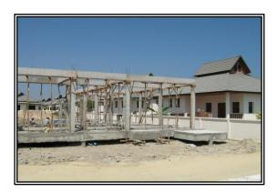
(<u>Remark</u>s: Some projects don't have the secondary ring beam to support the roof, only steel structure being welded to the steel from the pole. It's faster and cheaper but less strength)
