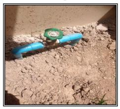
zoning water closet valve for bathroom and kitchen allows easier maintenance work. While maintenance, the system can be shut down and repaired accordingly.
